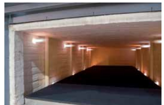
Furnace chamber with eight high-speed burners
