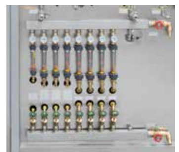
Cooling water distribution
