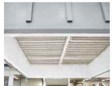
Heating elements in furnace hood
