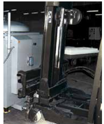
Slots under the furnace for the forklift forks
