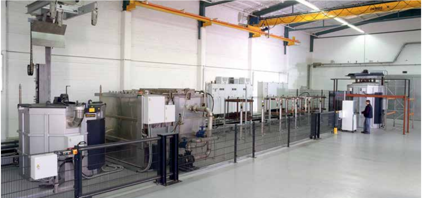
Fully automatic tempering system for aluminum with 2 pit furnaces, water bath, and 6 parking places
